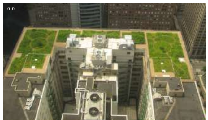
Green Roof in Chicago: en.wikipedia.org/wiki/Green_roof
